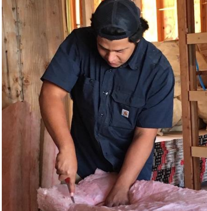
The Brenkle Court team has kept busy installing insulation.
