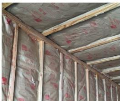
The Brenkle Court team has kept busy installing insulation.
