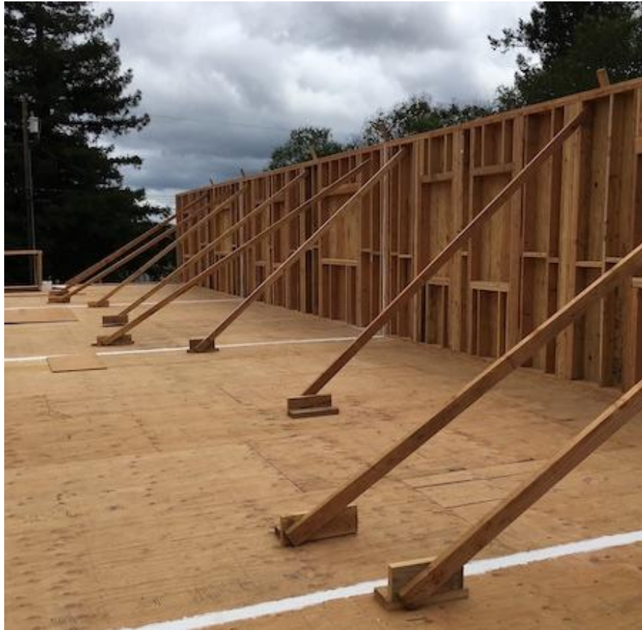
Framing has officially begun on the second floor!
