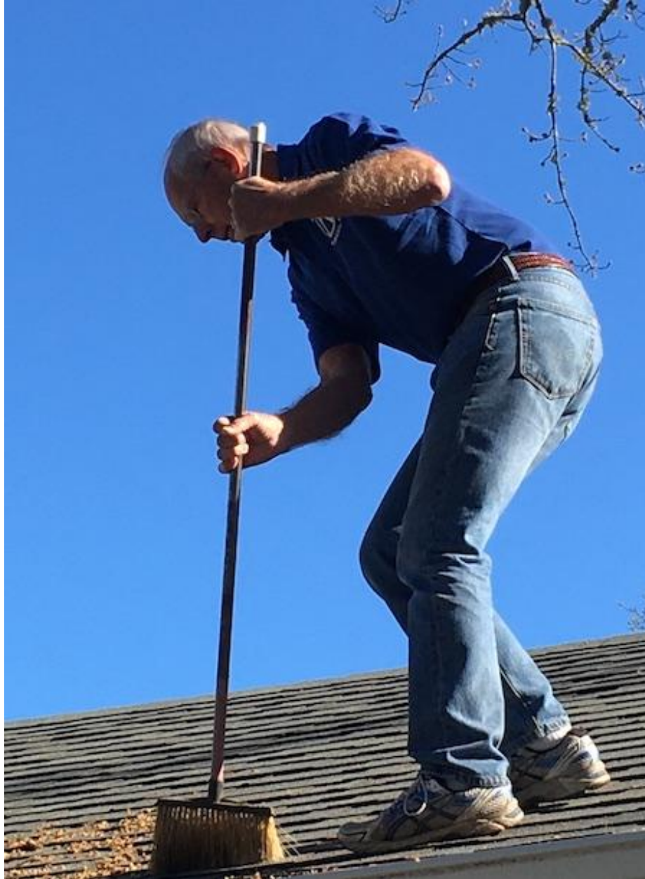
Bob Beckstrom cleaning gutters
